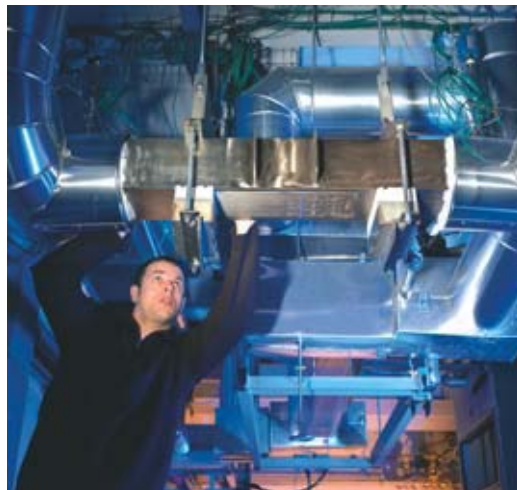
The CLAIRE loop, set up at the CEA Grenoble Center, is used in particular for gas-to-gas heat exchanger tests.
